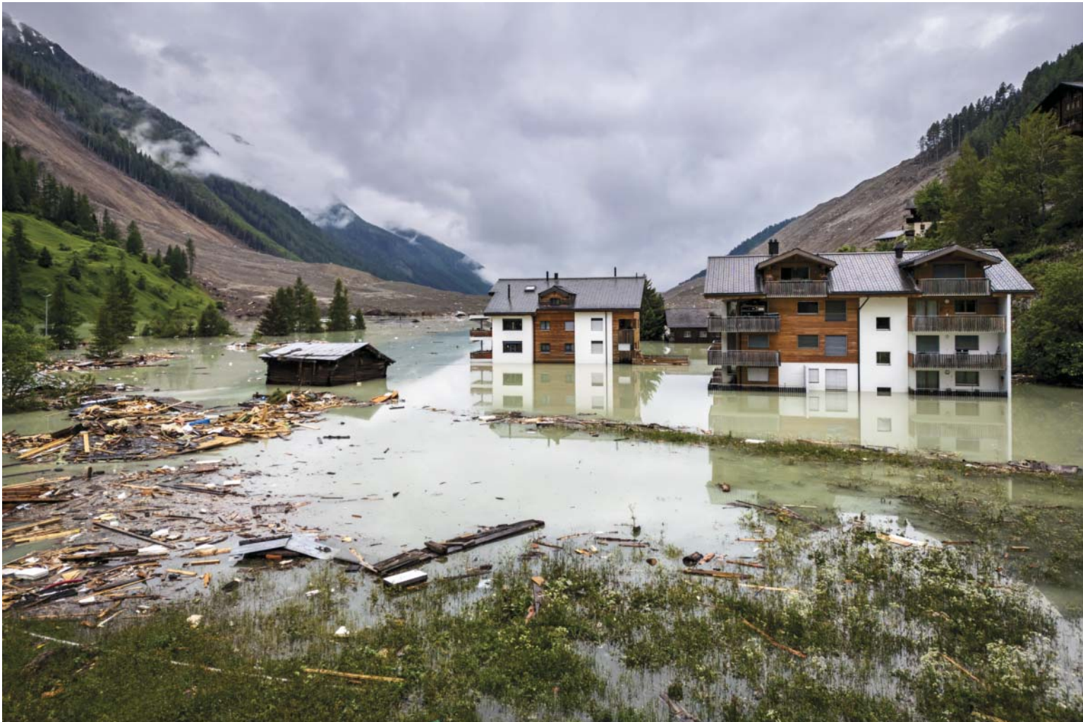
What remains of Blatten is beginning to flood following the collapse of the Birch glacier - 29/5/2025
